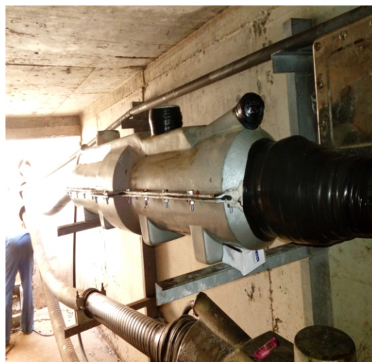
Combined Premoulded Joint
