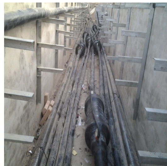
Combined Premoulded Joint
